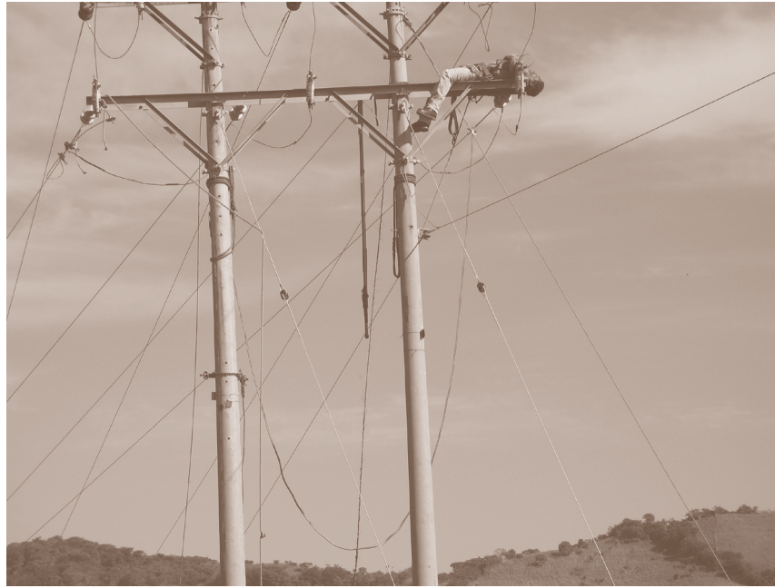
Subcontracted electricity worker in El Salvador, May 20, 2007.
