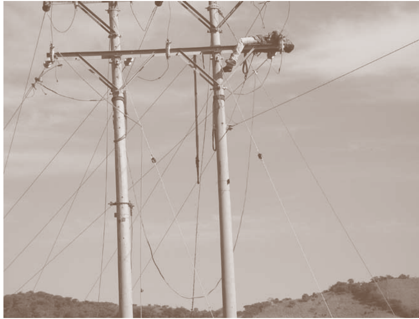
Subcontracted electricity worker in El Salvador, May 20, 2007.
