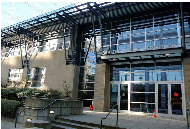
West Precinct, Seattle Police Department. Source: Abdar, WikiCommons
