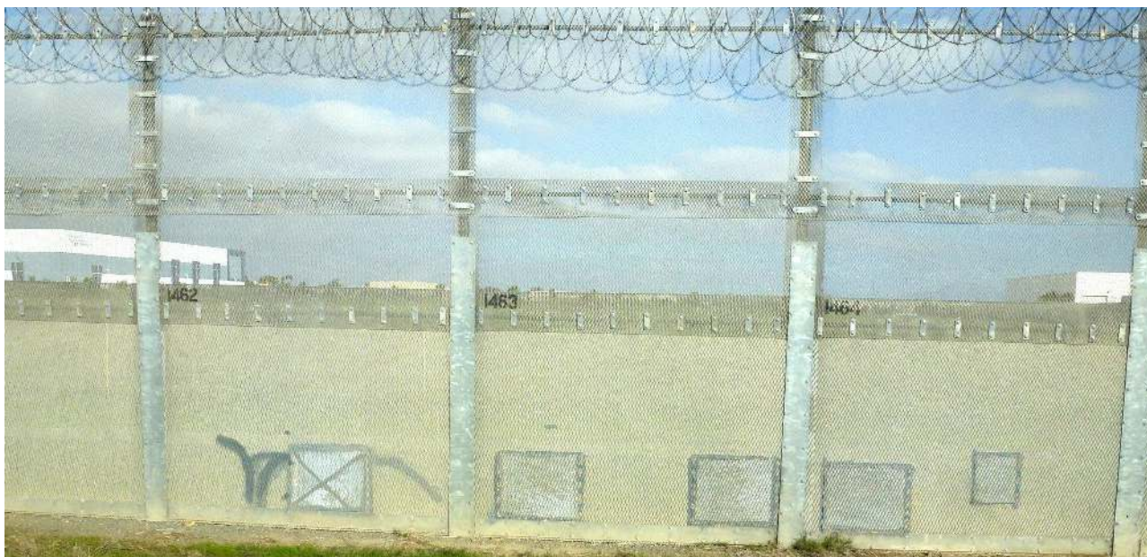
Patches in the San Diego border fence. (Credit: Adam Isacson)
